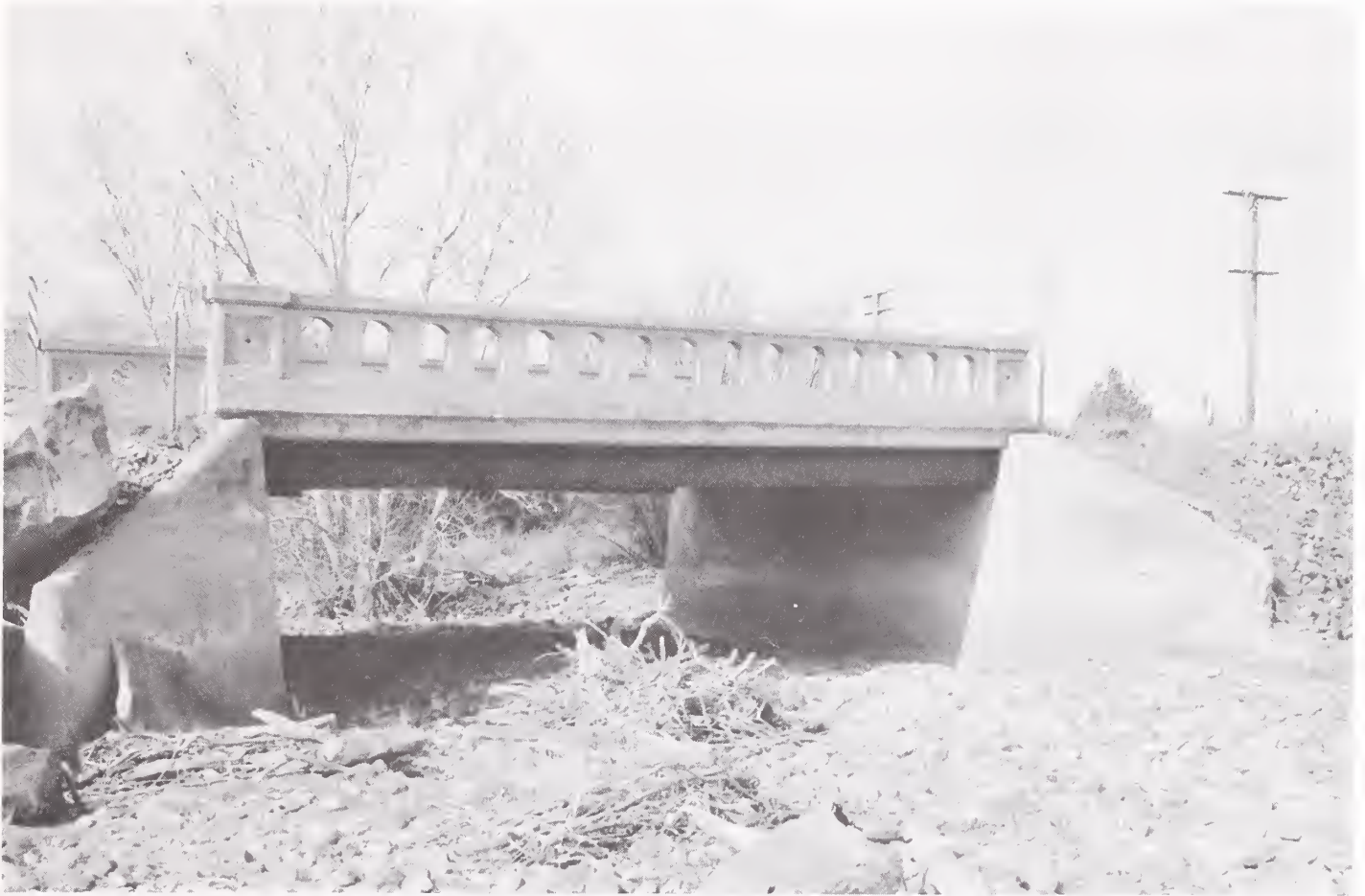
The Emigrant Creek Bridge, built in 1928.
